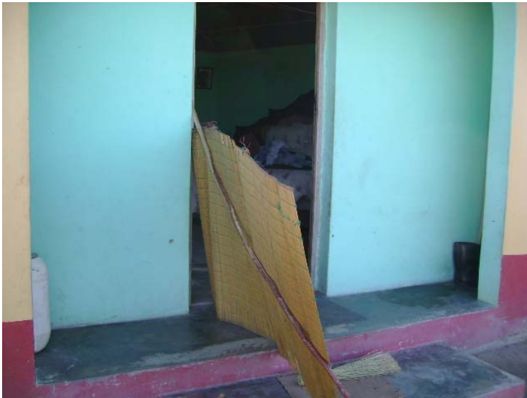
Picture 6. 4: Channelling air into a kitchen using the mat and stick technique
